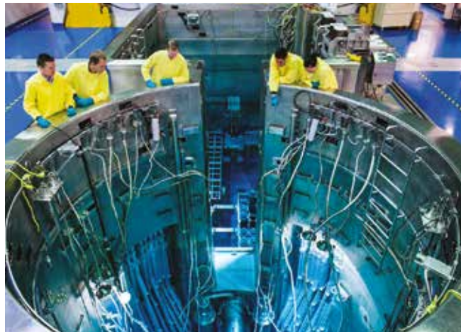
The OPAL Research Reactor, is one of the world's most effective multi-purpose reactors. The high energy beta particles from spent nuclear fuel immersed in water give rise to the distinctive blue glow called Cherenkov radiation. The OPAL Research Reactor is used for nuclear medicine, scientific research and industrial applications. Source: Australian Nuclear Science and Technology Organisation.
